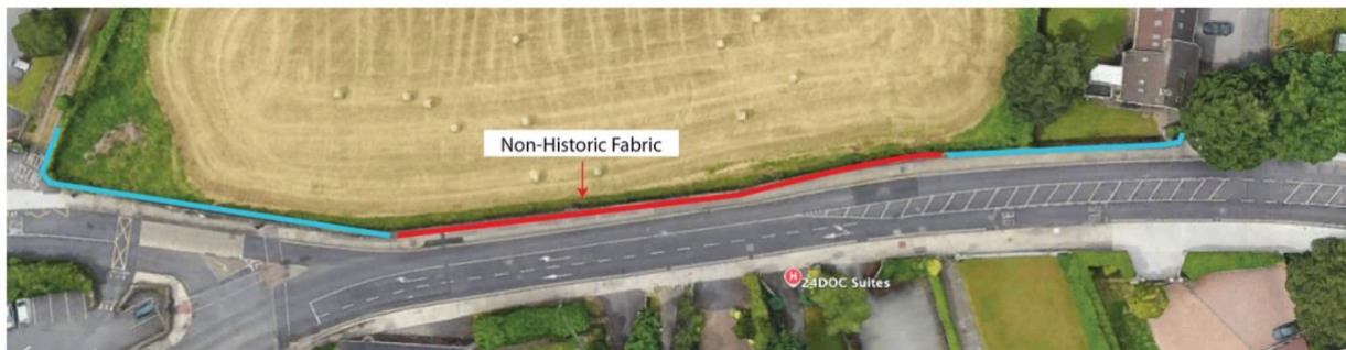
Figure 7 Indication of Non-historic Fabric of wall which has been re-built
