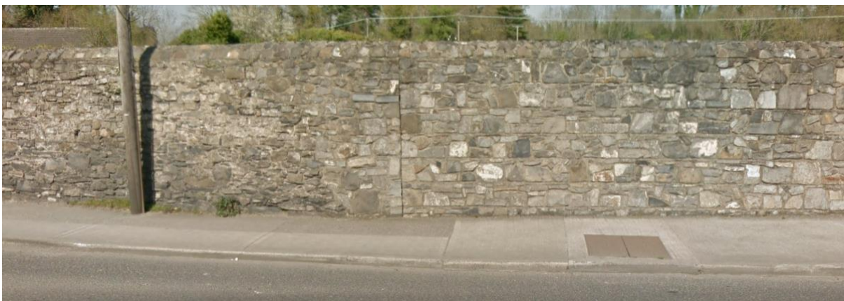
Figure 4 Elevation to Lucan Rd. Showing clear distinction in building methods.
